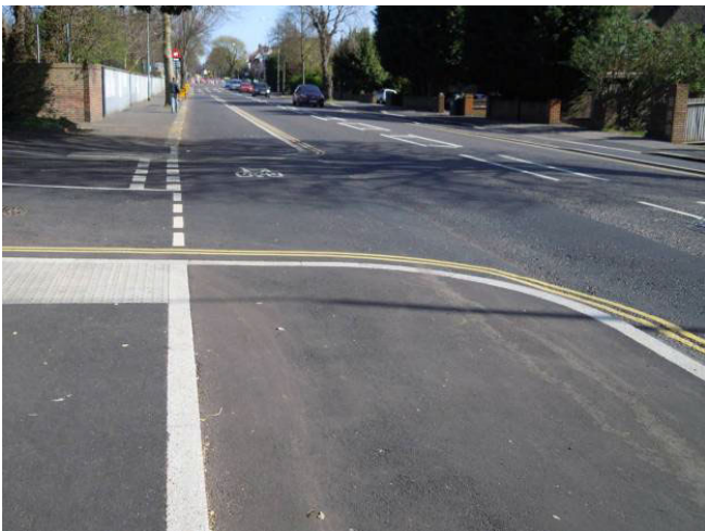
Details at side road crossing, minimised signs and marking to reduce street clutter were a key feature
