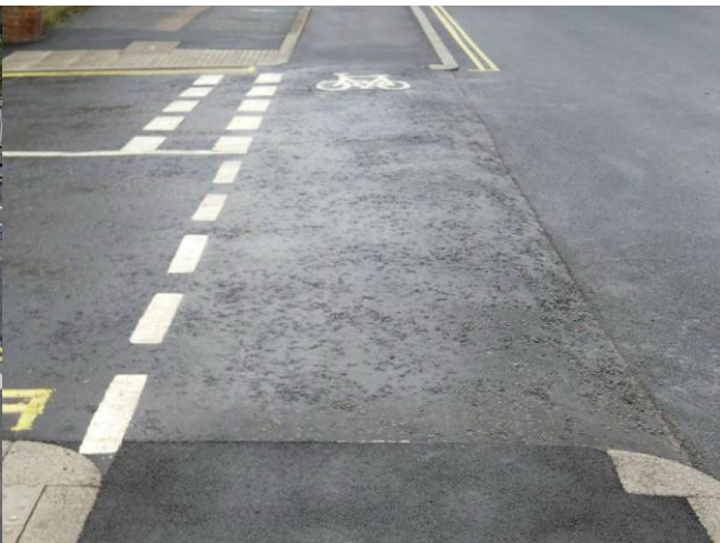
Details at side road crossing, minimised signs and marking to reduce street clutter were a key feature
